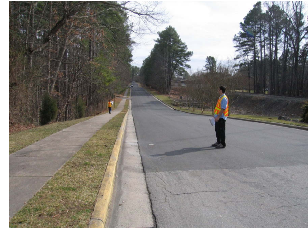
8. A3 - Village Dr. heading south east - RR on west side. Bike connection will avoid RR ROW.
