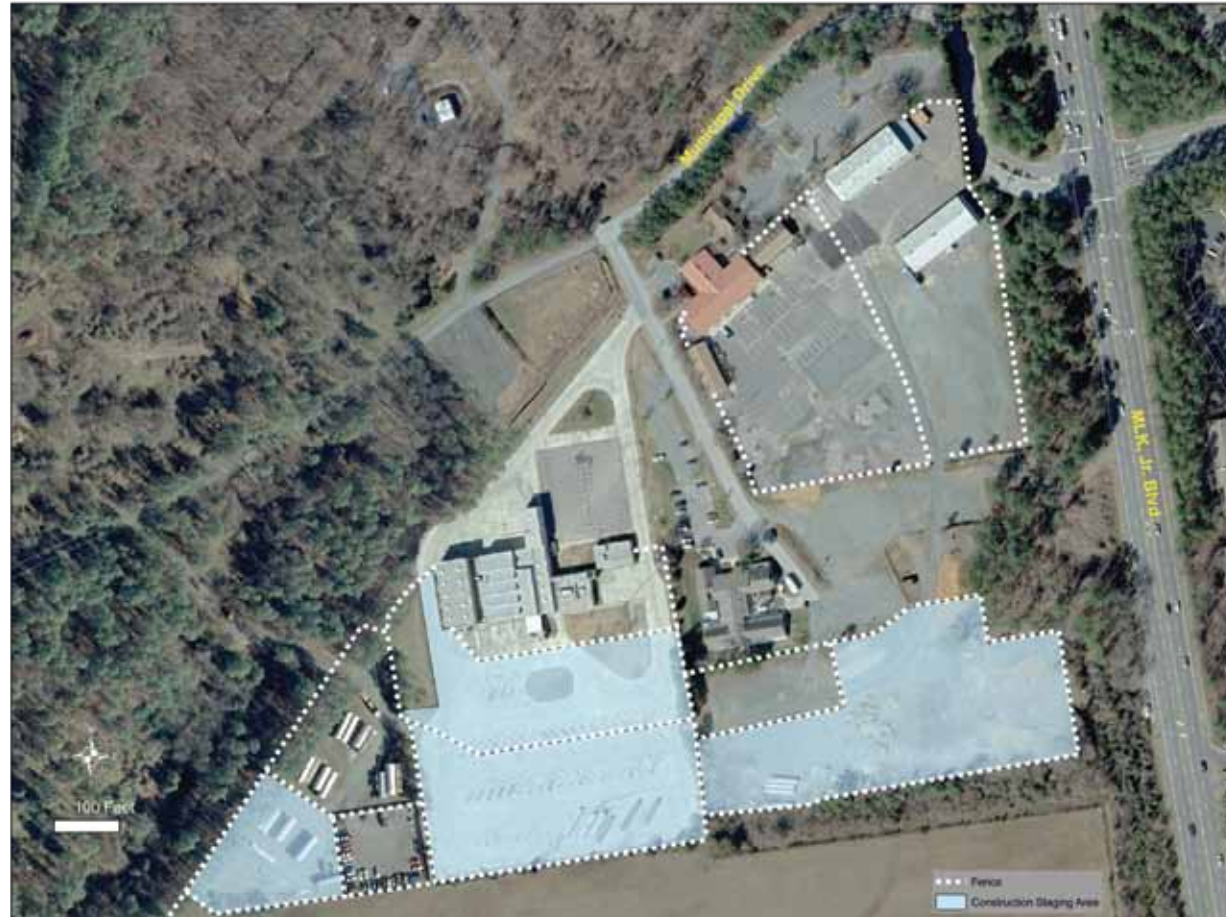
Exhibit 14. Site storage and construction staging areas
