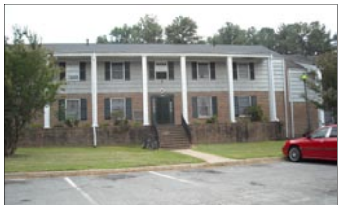
Housing stock in Chapel Hill is in overall good shape, but there are some older apartment complexes like the Colony Apartments (above) that are noticeably in disrepair.
