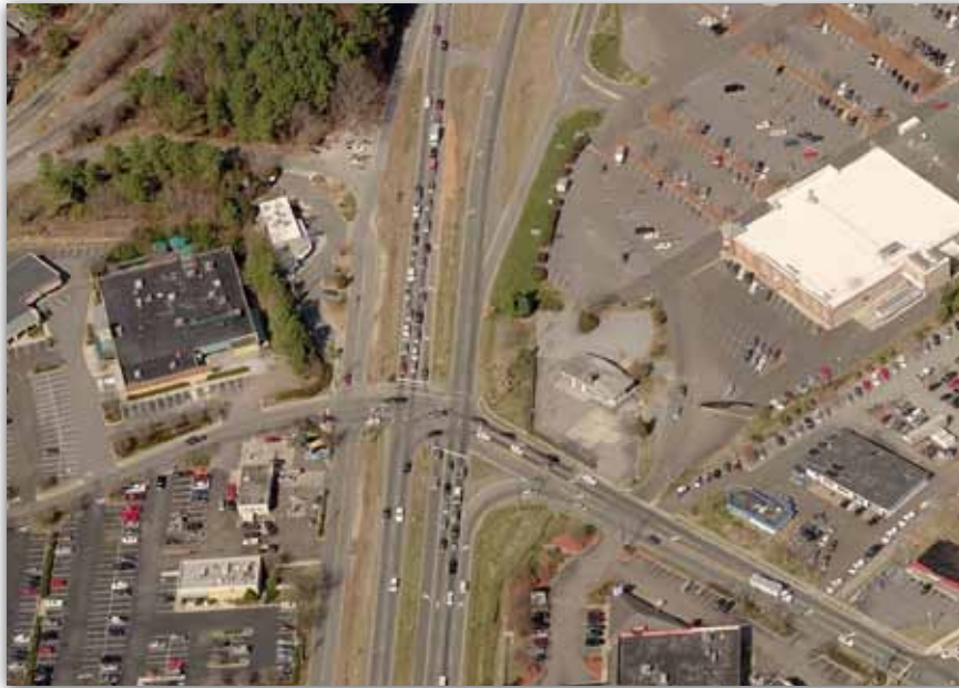
Fordham Boulevard - Ephesus Church Road Intersection
