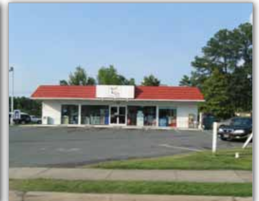
Out-parcel commercial buildings
