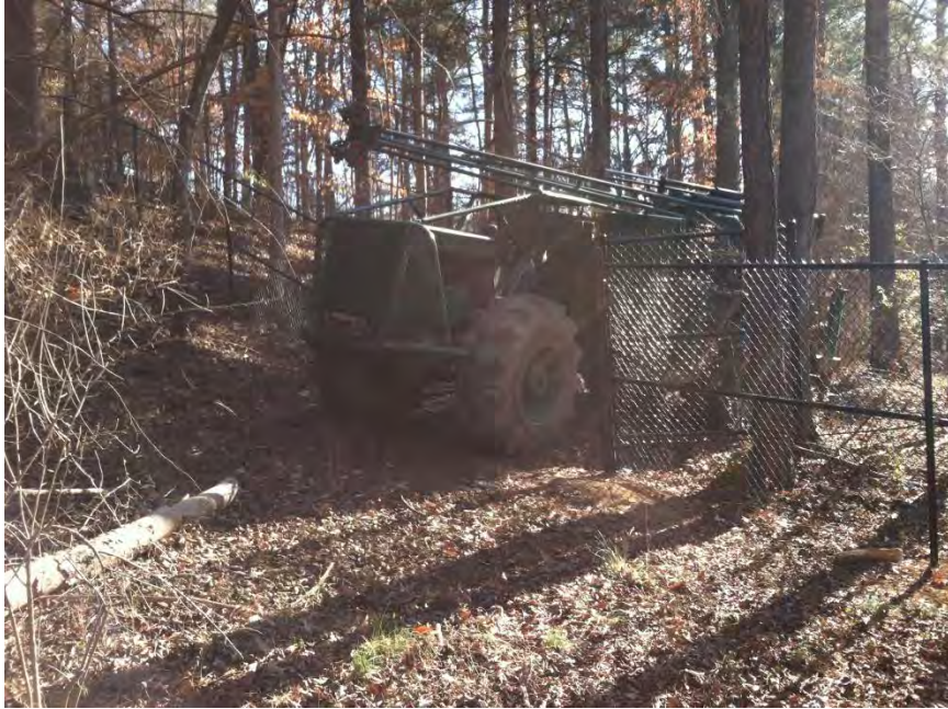
Drill Rig and fence gate
