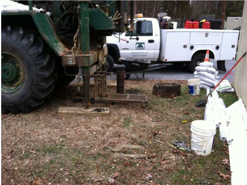
Attempted location for MW-5 in north
