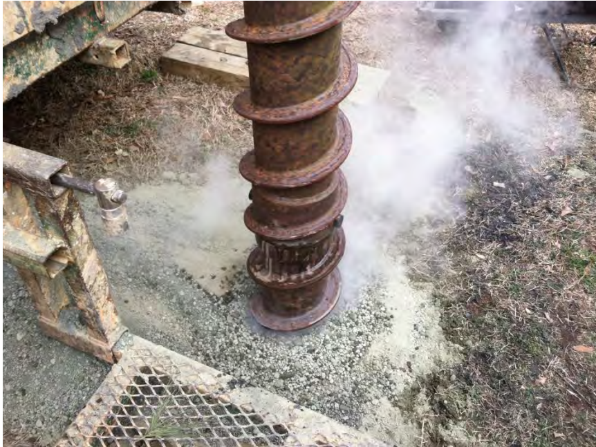
MW-5 encountered soils ~25-30 ft bgs
