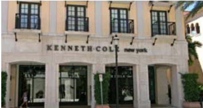
Arcades, balconies, and bays are all responses to south facing solar orientation
