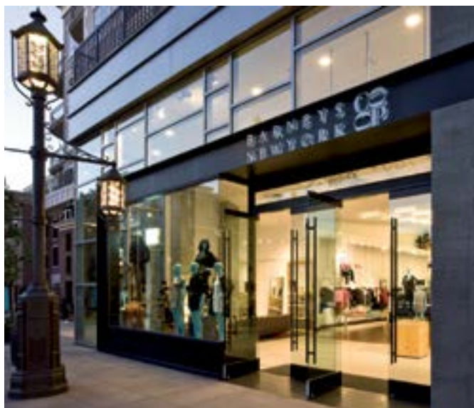
Spilled light creates a welcoming, safe public realm
