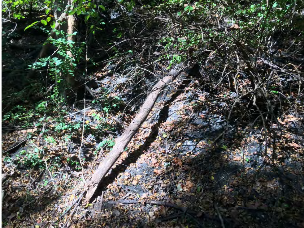
Photograph 3: CCP exposed at the surface along the central portion of the embankment .
