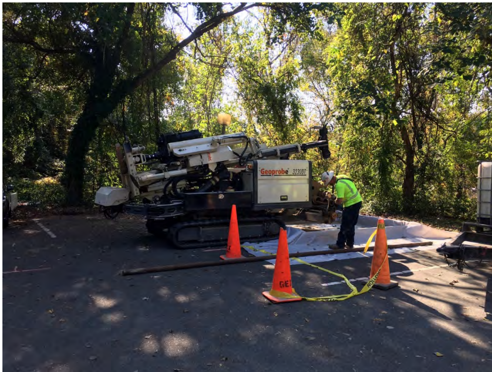
Photograph 9: View of the decontamination pit.
