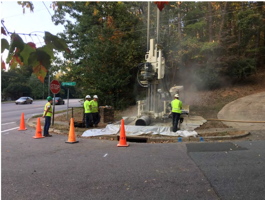
Photograph 6: Installation of MW-5. View is to the north.
