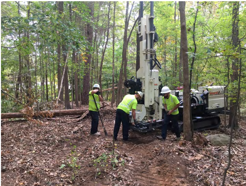
Photograph 8: Installation of MW-7. View is to the east.
