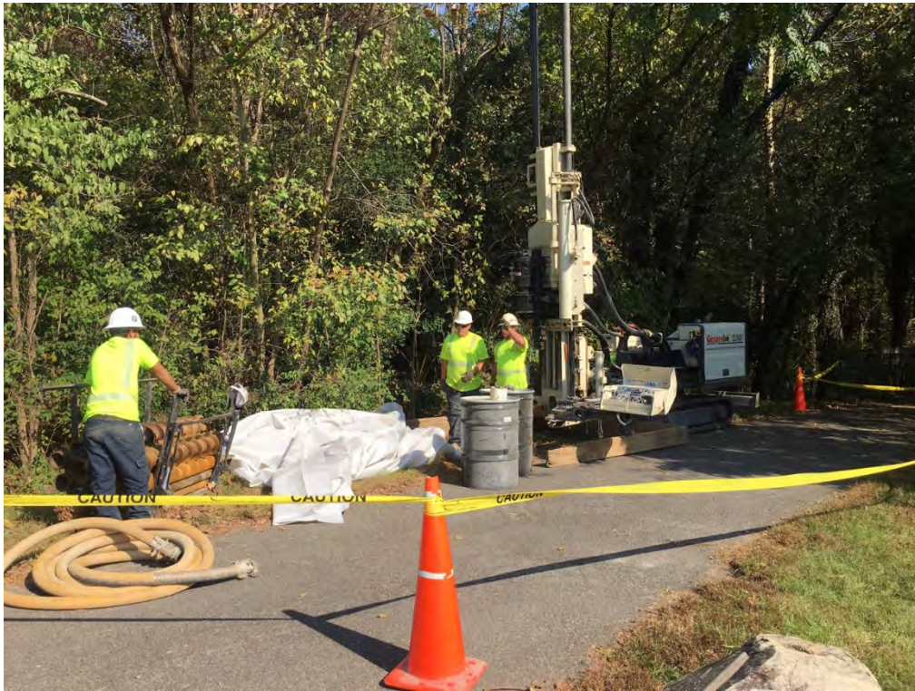
Photograph 7: Installation of MW-6. View is to the northeast.
