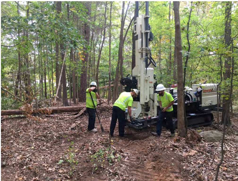
Photograph 8: Installation of MW-7. View is to the east.
